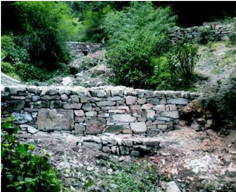
Check walls on a stream for water conservation
